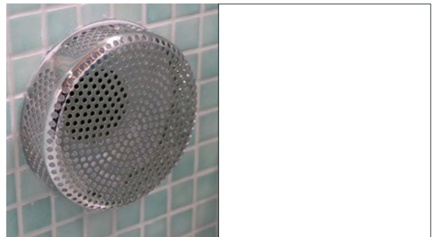
- Suction fitting (AquaFun 4.0): d63 port - Suction fitting (Spa Massage Pak): d50 port = Jet pump suction side
