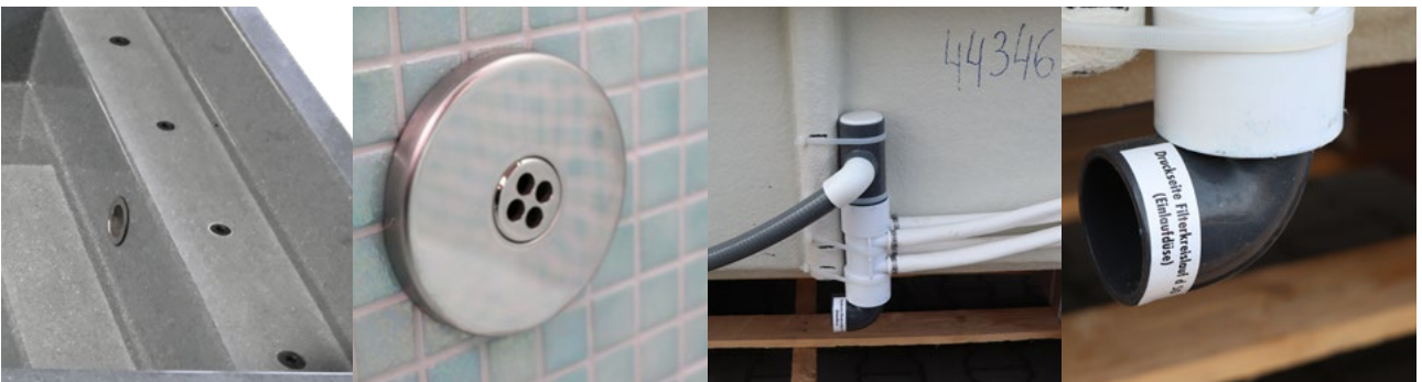
- 4x spring inlet and inlet nozzle d50 port = filter pump, pressure side
