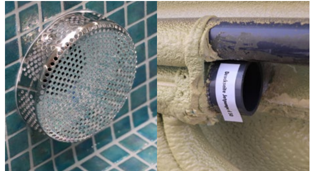
- Suction fitting: d50 port = 1.0 kW jet pump, suction side
